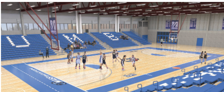
This summer, crews put in a new hardwood floor and bleachers at the Clark Center gym and installed new lighting and Wi-Fi. Volleyball, basketball, and intramurals are breaking it in this fall.
